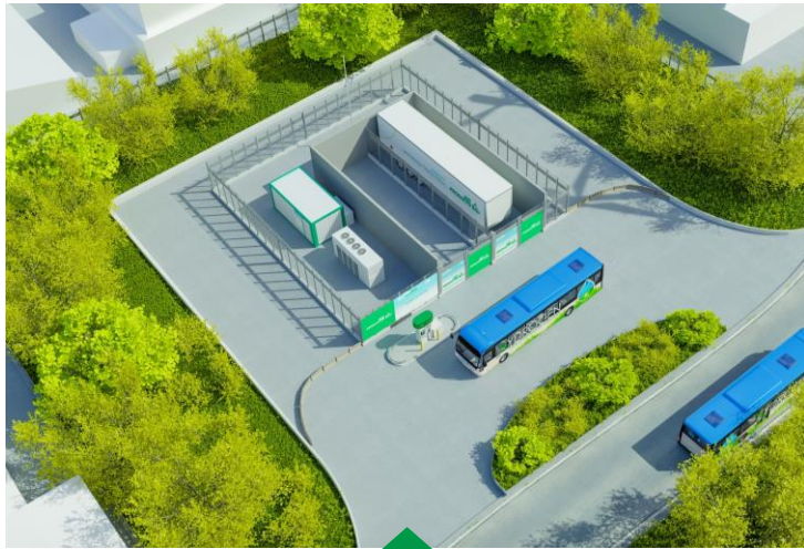
Gas based Station (350 bar) Up to 1 ton/day Buses Small Fleets
