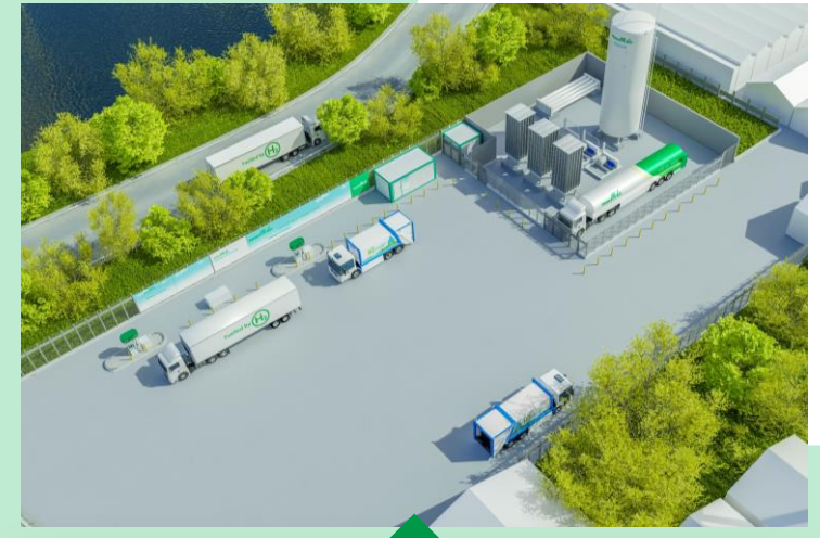
Multimodal Station (350 & 700 bar) Up to 5 tons/day Buses & HDV Fleets
