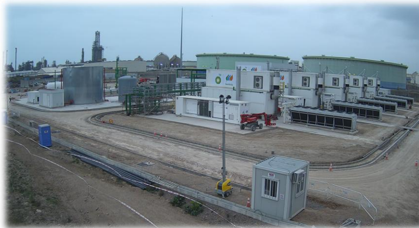
Containers arrival at the site, Q3 2025
